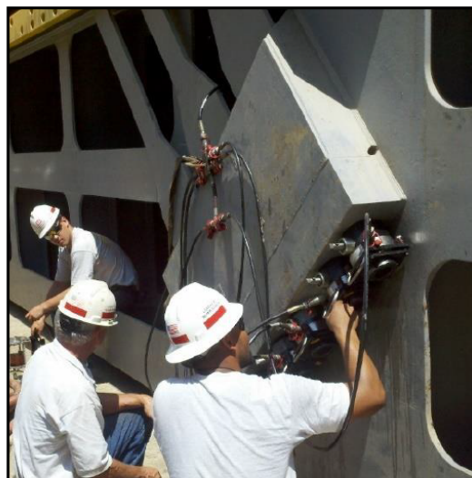
Figure 2-18: Multiple nut tensioning mechanism using multiple stud tensioners
