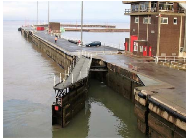
Bristol Portbury Lock gate (42.7 m) (photo F. de Crescenzo)
