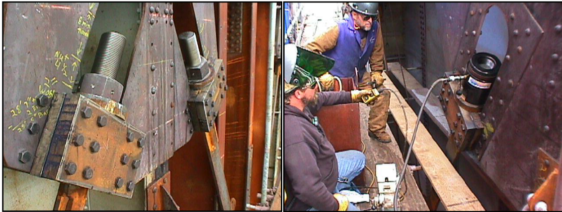
Figure 2-17: Diagonal with threaded ends and large nut (115-mm diameter) and with hydraulic tensioner attached (right)
