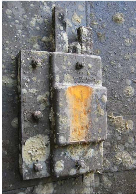
Lower fixed thrust block
