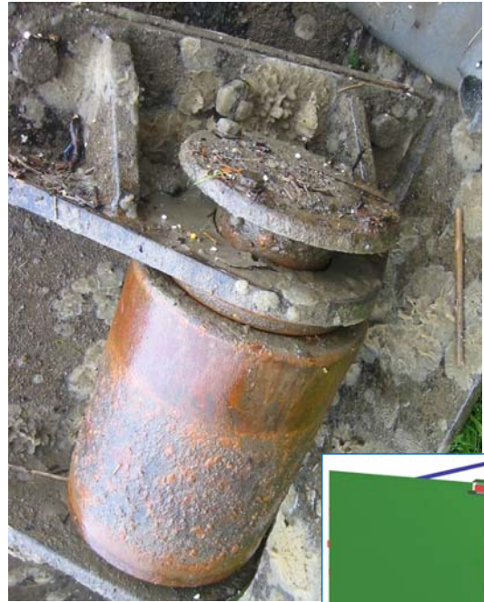
Rolling thrust block
