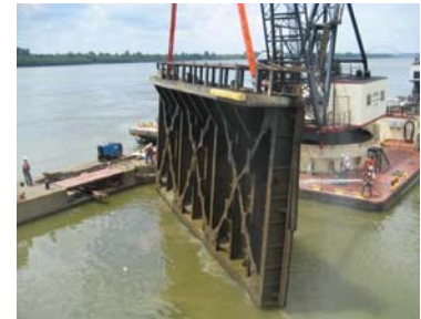
Ohio River Lock 52
