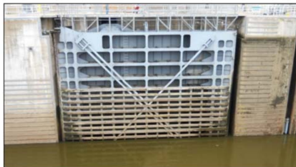
Figure 6-16: Typical fendering (Lock 19, Mississippi River)
