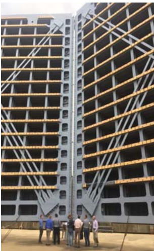
Louisville Lock miter gate
