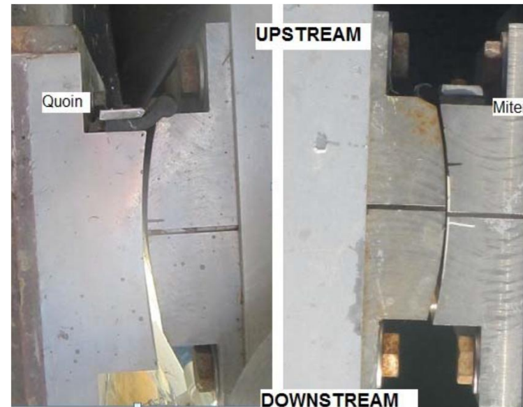
Contact blocks with Rubber Seals
