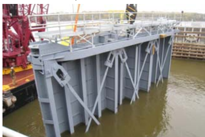
Mississippi, Lock & Dam 21, USA
