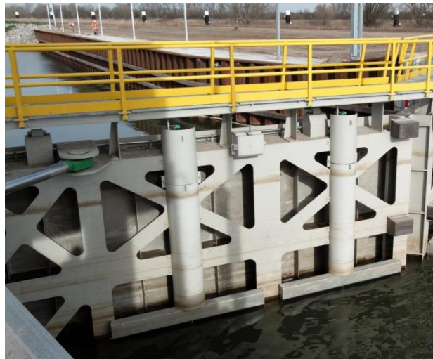
Structural framing and Machinery Protection
