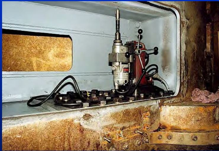
Temporary repairs, new cover plate
