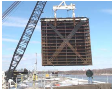
Ohio River Lock 2
