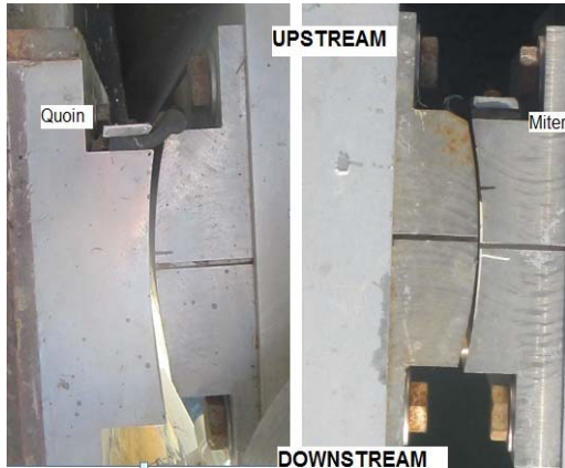
Figure 2-16: Mechanically adjustable quoin blocks of The Dalles mitre gate, USA
